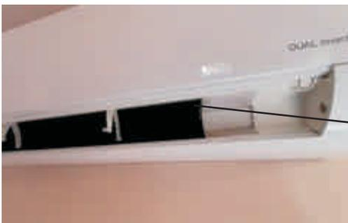
First step is to Power off the entire AC Unit, then you need to remove the AC Air swinging flaps with a screw driver
