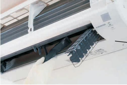
Then clean the surface near the Air Blower, should have no dust, grease, or any residual, use brush and moist cloth for optimal cleaning.
