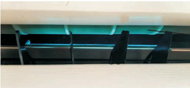
When finally assembled inspect and power on the unit, this is how the UV lights installed work when in operation, it focus the UVC light on to the AC Air blowers this killing biological contamination as well cleans room air.
